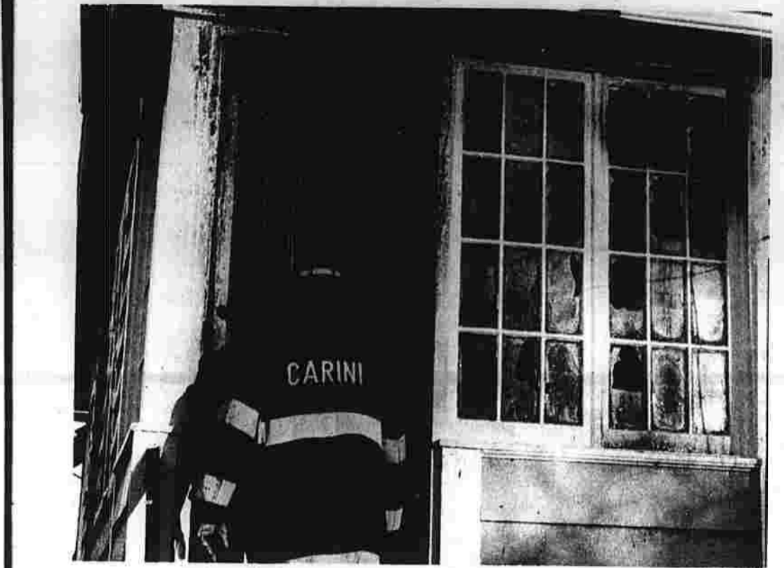
Town Firefighter Edward Carini enters the scorched back porch of the home of Kenneth and Joan Burnett at 84 Benton St. immediately after a fire there Thursday afternoon. The fire caused extensive damage to the back porch and the kitchen of the home. (Herald photo by Pinto)
